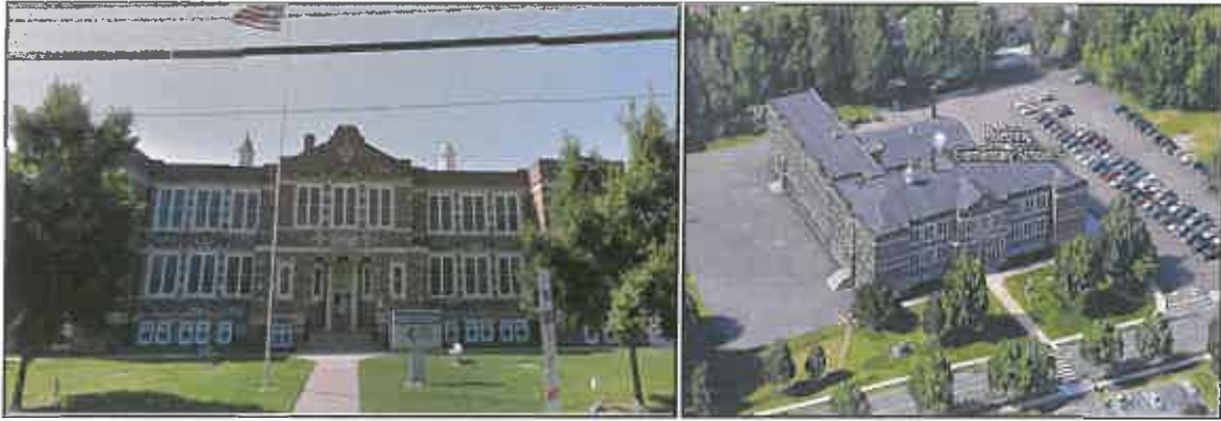
Photos 1 and 2. Roebling Elementary School, 1330 Homberger Avenue, Roebling.
