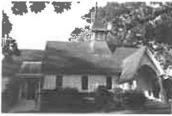
Main Church Building Roy, J. (1985). Providence Presbyterian Church of Bustleton . National Register of Historic Places Inventory Nomination.
