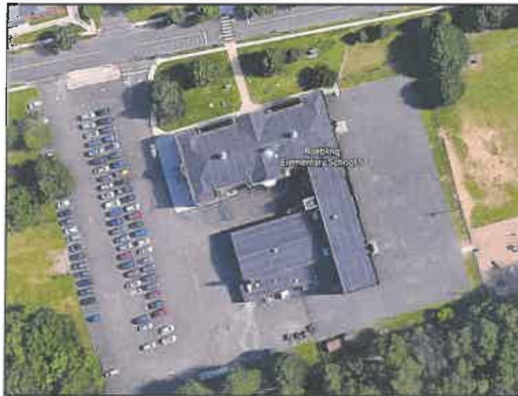
Photo 3. Aerial View of Roebling Elementary School.
