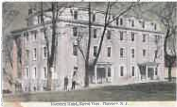
Florence Hotel. Source: West Jersey History Project
