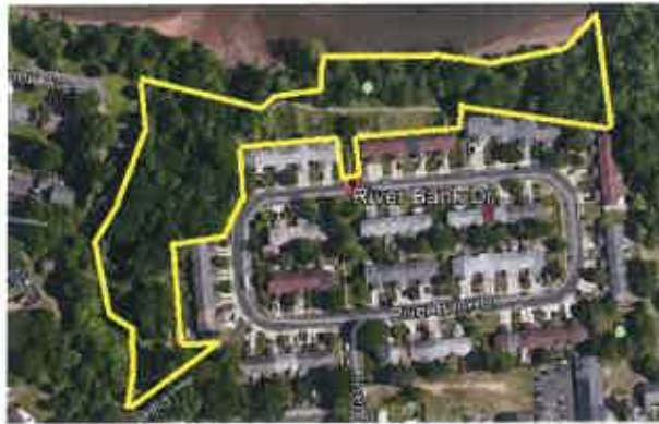
Site 6. River Bank Drive Park and Walkway.
